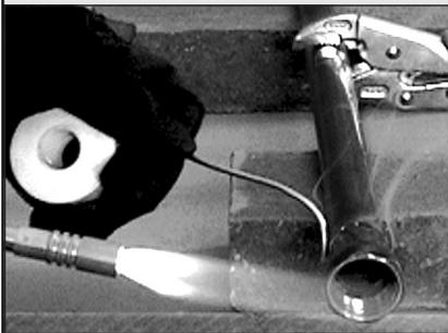
**NOTICE:** Do not solder pipes while they are attached to the water heater. The water heater's inlet and outlet connections contain non-metallic parts which could be damaged. The proper way to connect the water heater to copper water pipes is as follows:
