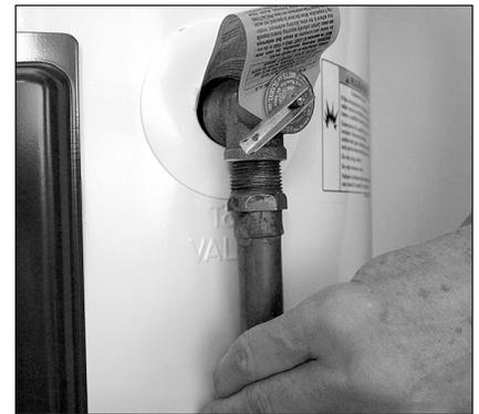
Figure 15 - The T&P Relief Valve discharge pipe must be installed properly and piped to an adequate drain.
