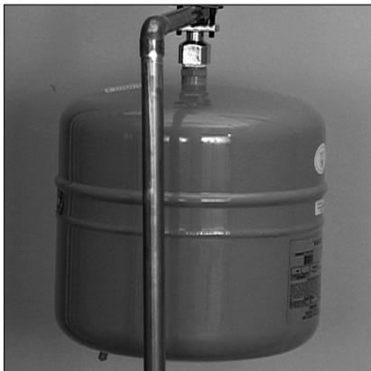
Figure 18 - The Thermal Expansion Tank should be pressurized with air to match the home's incoming water pressure.
